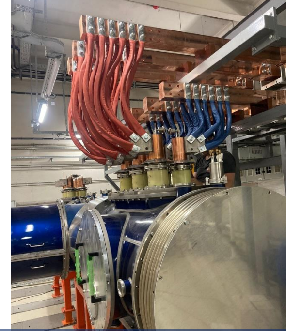
Power lines are connected
