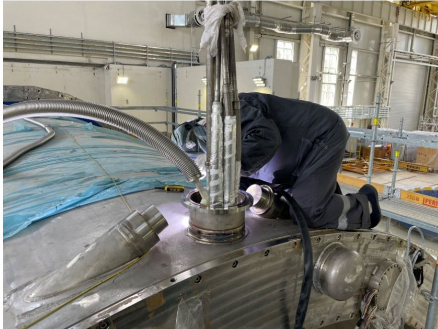
Figure 2. Preparation of the chimney node by JINR specialists
