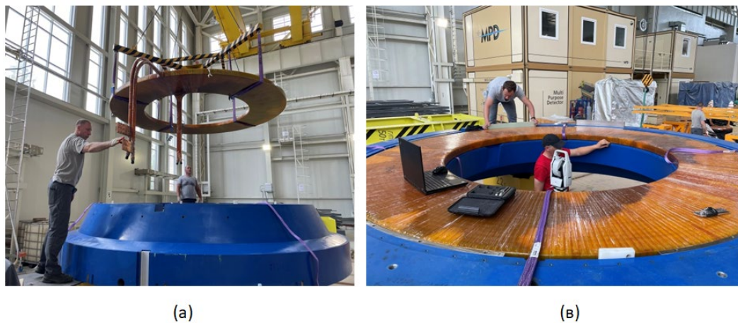
Figure 3. Assembly of correction coils, where (a) is the coil-pole assembly, and (b) is the alignment measurement.
