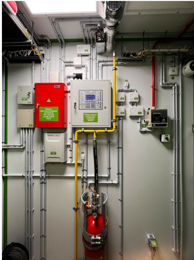
Fig 3.10.3. Fire automation of extinguishing system
