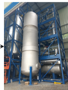
Distillation: remove radioactive impurities
