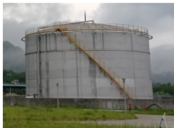
5000 m 3 LAB tank
