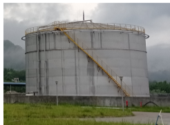
5000 m 3 LAB tank
