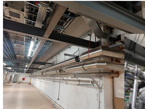
Cryogenic LHe, LN 2 , warm straight and return pipelines
