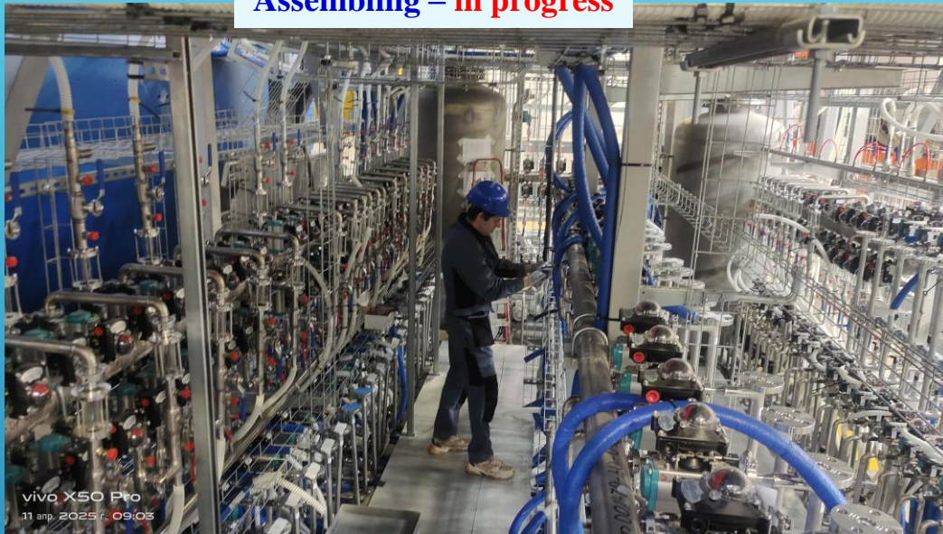
Assembling – in progress
