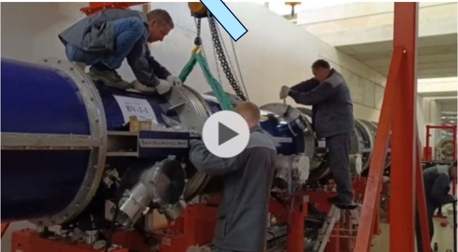
Last flange. Vacuum pumping of the W-arc is started. Sept 12, 2025 Cooling of the cryo-magnetic system has been started 14 Sept 2025
