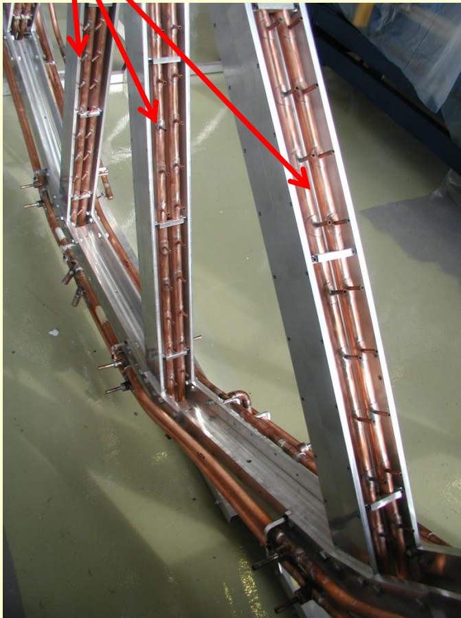
Pipes for ROC electronics cooling
