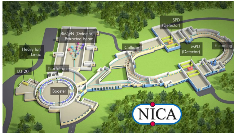
Figure 33: Layout of the NICA collider with SPD at the south collision point..
