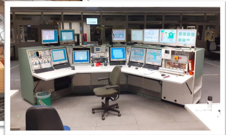
MLL Control Room
