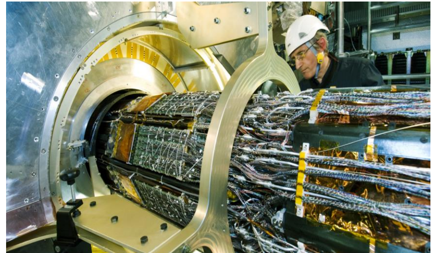
Michal Tomasek from our group during the installation of the Pixel Detector in the ATLAS underground experimental hall
