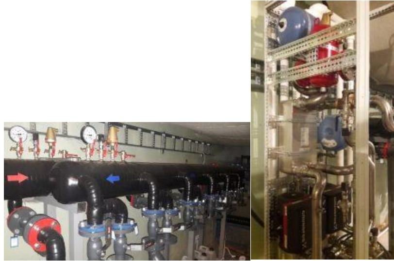
Fig.13. Elements of the GOVORUN supercomputer liquid cooling system: the collector, the rack with a pump and a heat exchanger.
