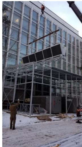
Fig. 12. Installation of a dry cooling tower.
